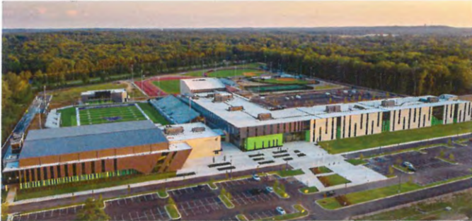
LITTLE ROCK DISTRICT Southwest High School
