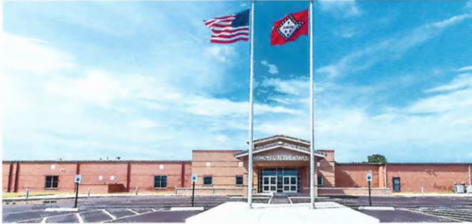
ARMOREL SCHOOL DISTRICT K-4 Building Addition & Renovations
