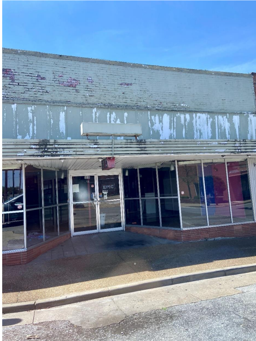
Figure 67: Abandoned Building Downtown
