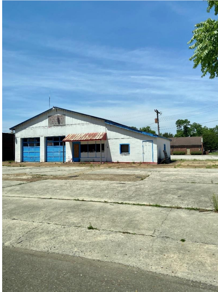
Figure 64: Abandoned Building and Lot
