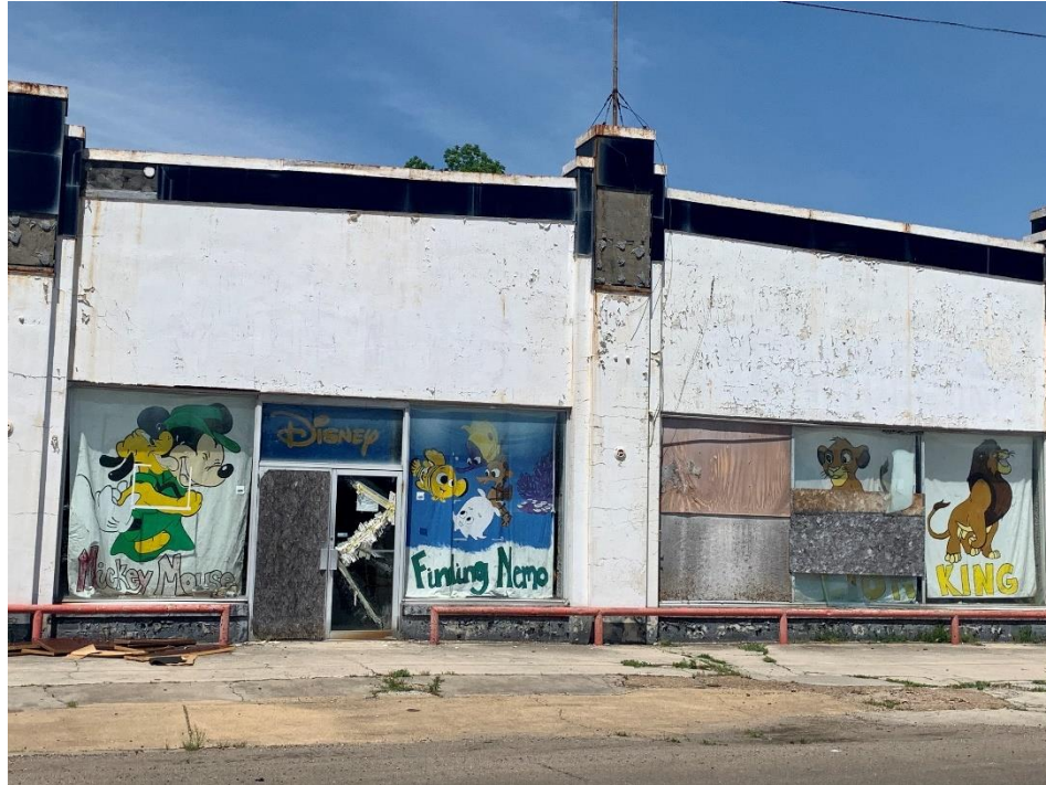
Figure 61: Abandoned Building Behind Courthouse
