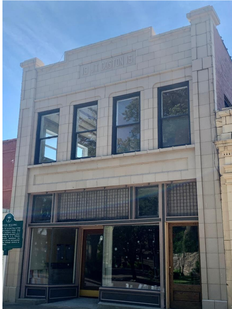
Figure 66: Coston Building Downtown
