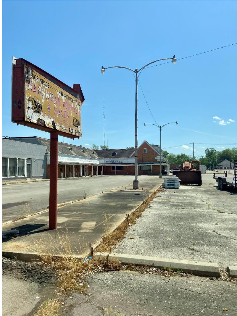
Figure 62: Dilapidated Lot Behind the Courthouse
