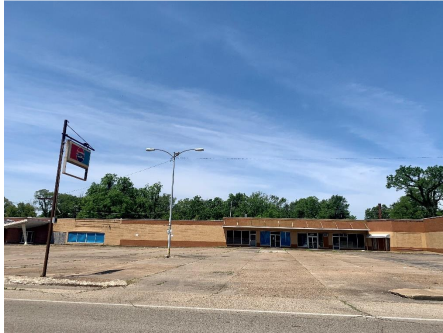
Figure 63: Abandoned Former Hotel
