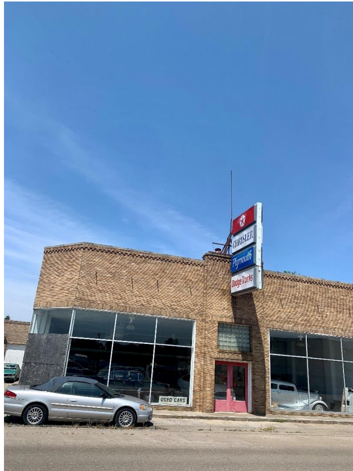
Figure 54: Old Car Dealership Near Radio Station
