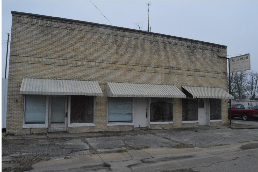
Figure 24: Exterior of KOSE 860 AM Radio Station
