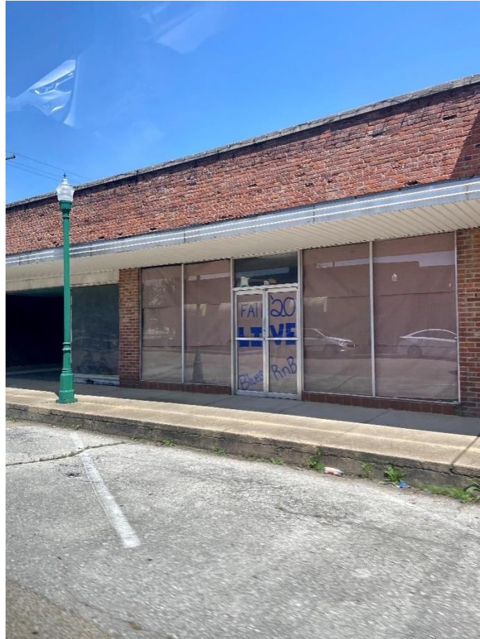
Figure 65: Abandoned Building Downtown
