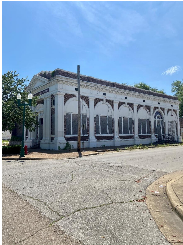
Figure 69: Abandoned Historical Building
