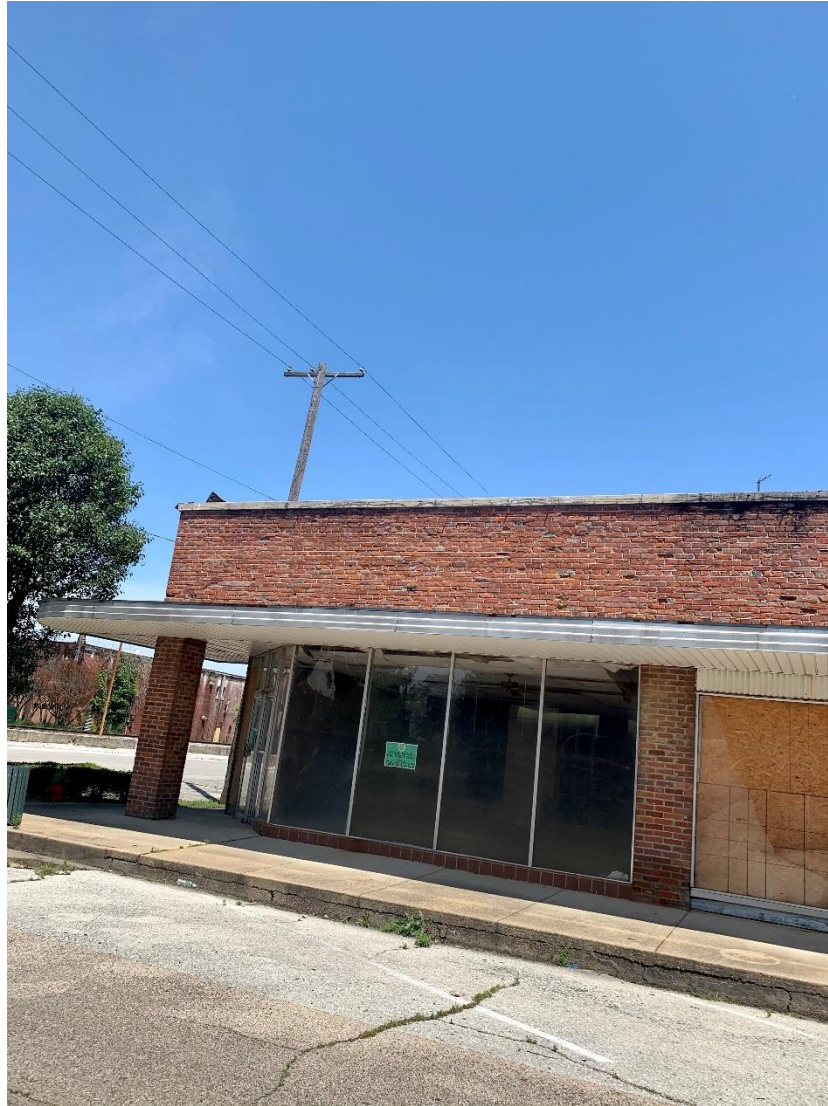
Figure 68: Abandoned Building Downtown
